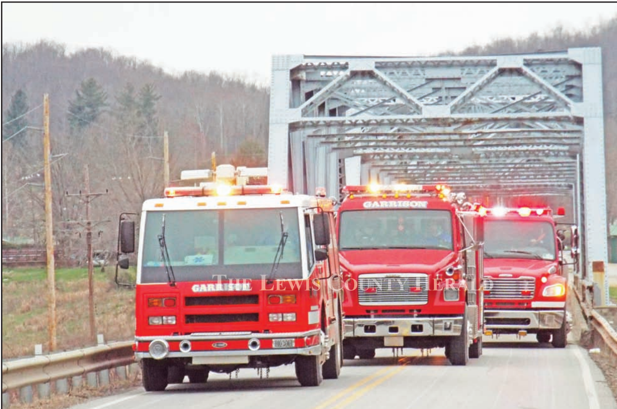
Karen Killen/LEWIS COUNTY HERALD Fire trucks from the Garrison Volunteer Fire Department cross the Blue Bridge a final time before the structure was closed for a replacement project. Safety concerns are paramount concerning traffic detours while the bridge is closed.
